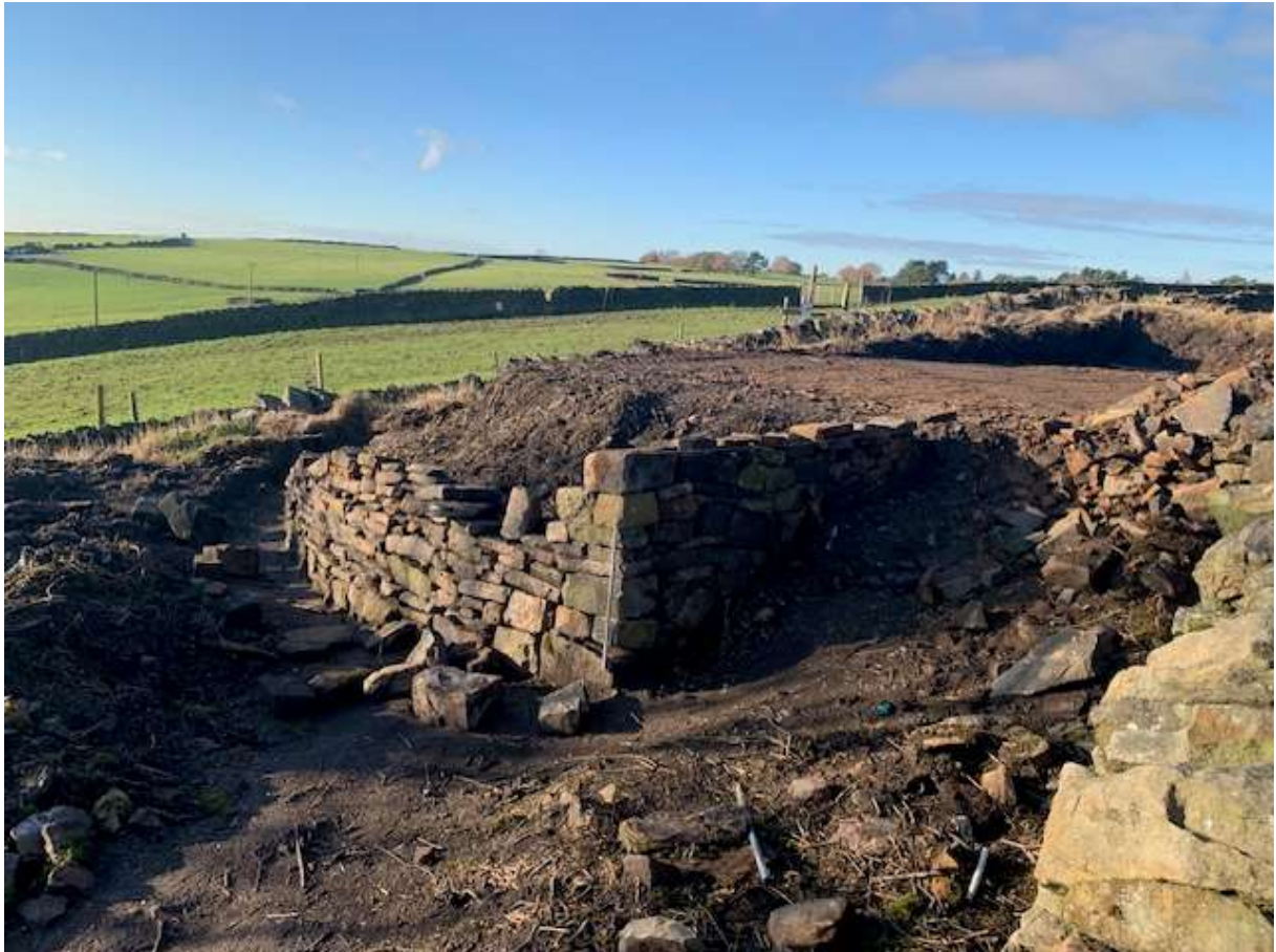
Figure 6 – Feature wall constructed from uncovered stone within the site
