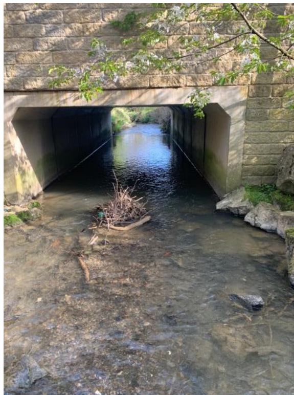
Photograph 4 – culvert further downstream of site.
