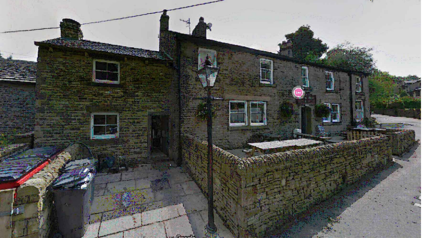
Site photo - West (front) elevation
