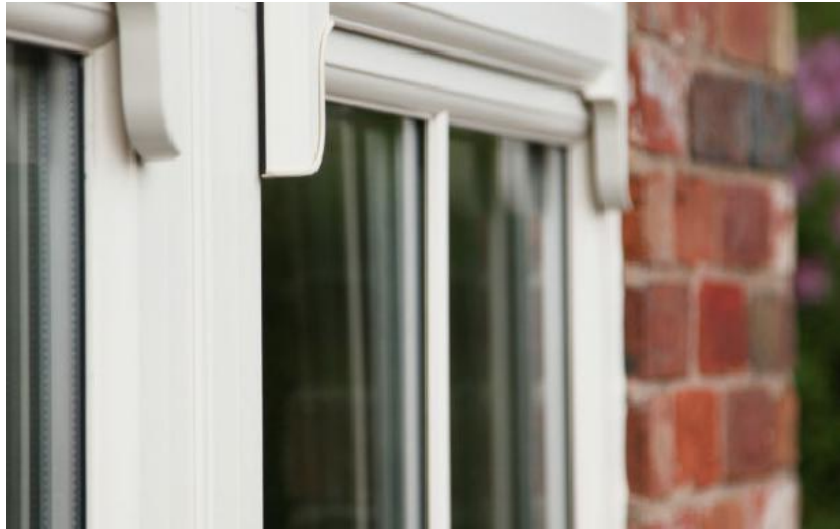
Proposed uPVC window to match existing style with traditional horn detail. Colour to match existing
