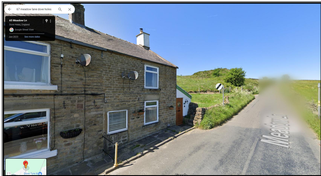
Figure 7 : Terraced block adjacent #67
