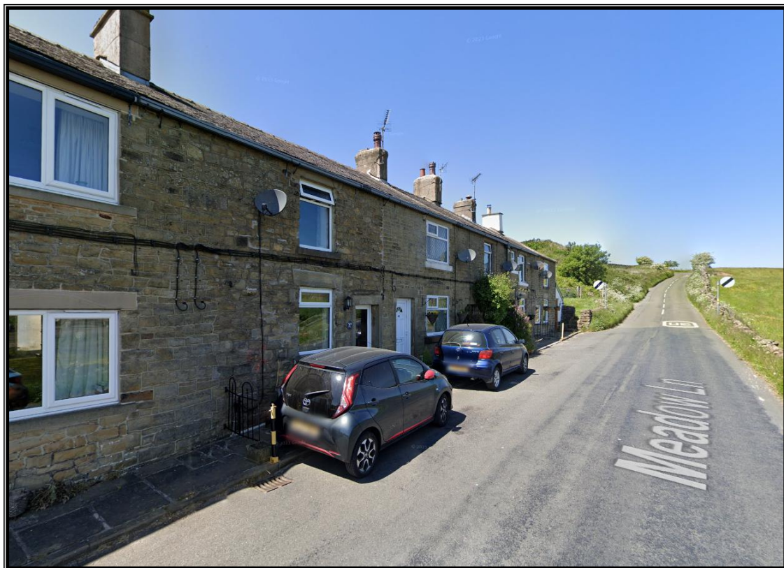
Figure 5 : Terraced block adjacent #67
