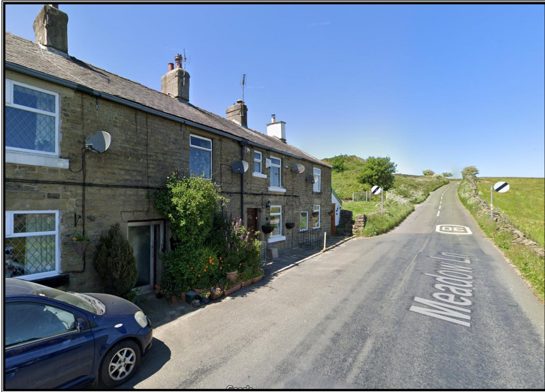
Figure 6 : Terraced block adjacent #67
