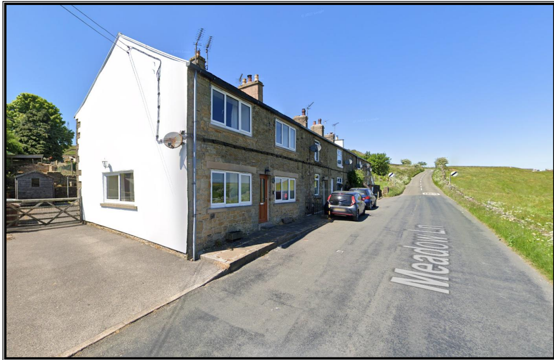
Figure 4 : Terraced block adjacent #67
