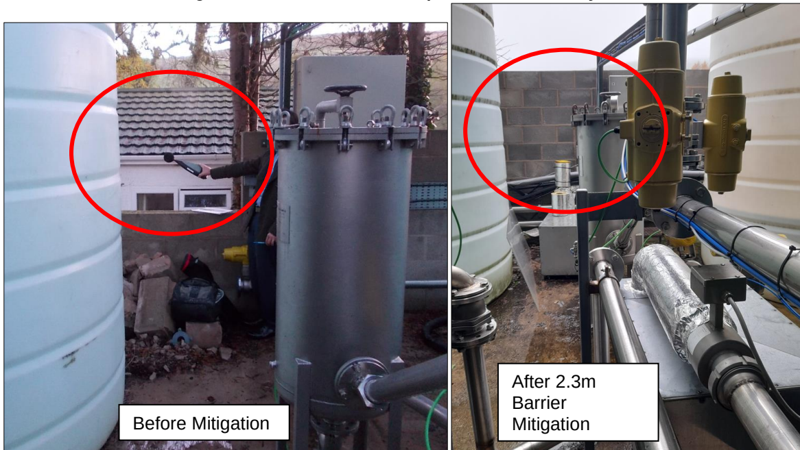
Image 2.2 – Before and After – Improved Site Boundary Noise Barrier
