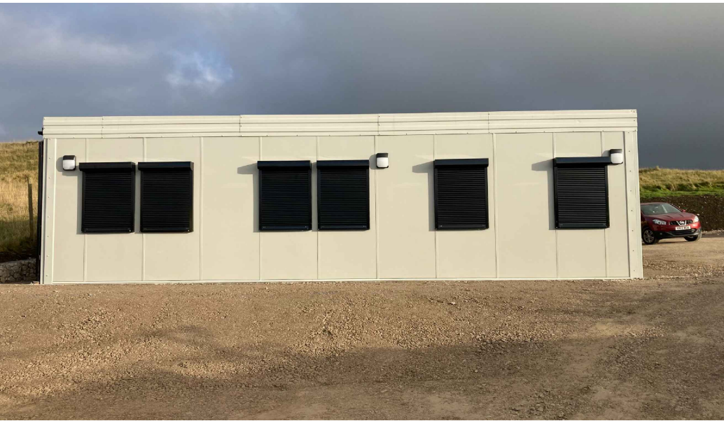
ELEVATION B EXISTING PHOTO REFERENCE
