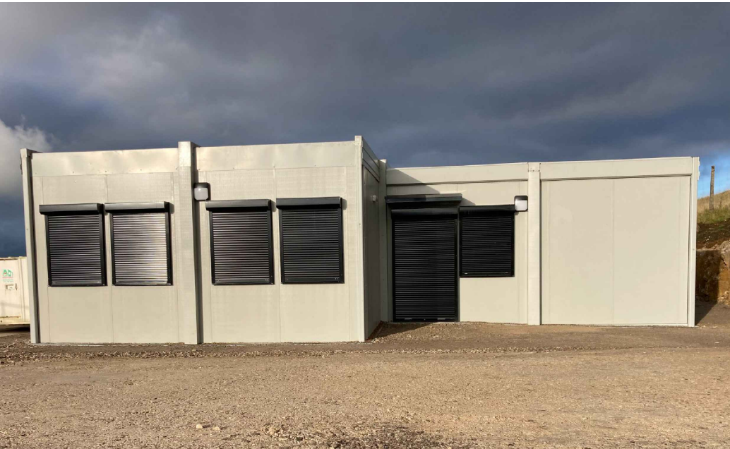
ELEVATION A EXISTING PHOTO REFERENCE
