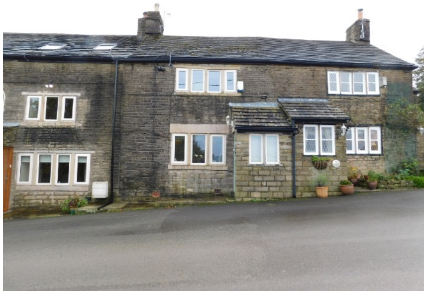
Front view of the property - 23 Back Lane
