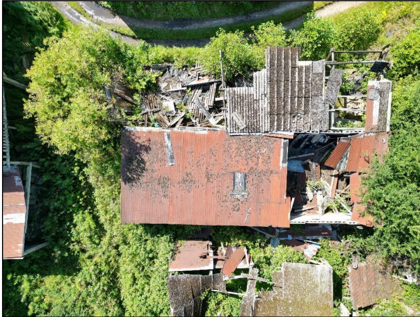
Photograph 17 showing the roof of Building 5
