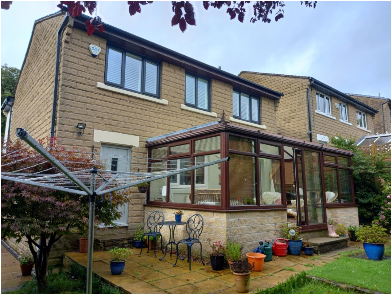
REAR ELEVATIONS OF 33, WOOD GARDENS, HAYFIELD.
