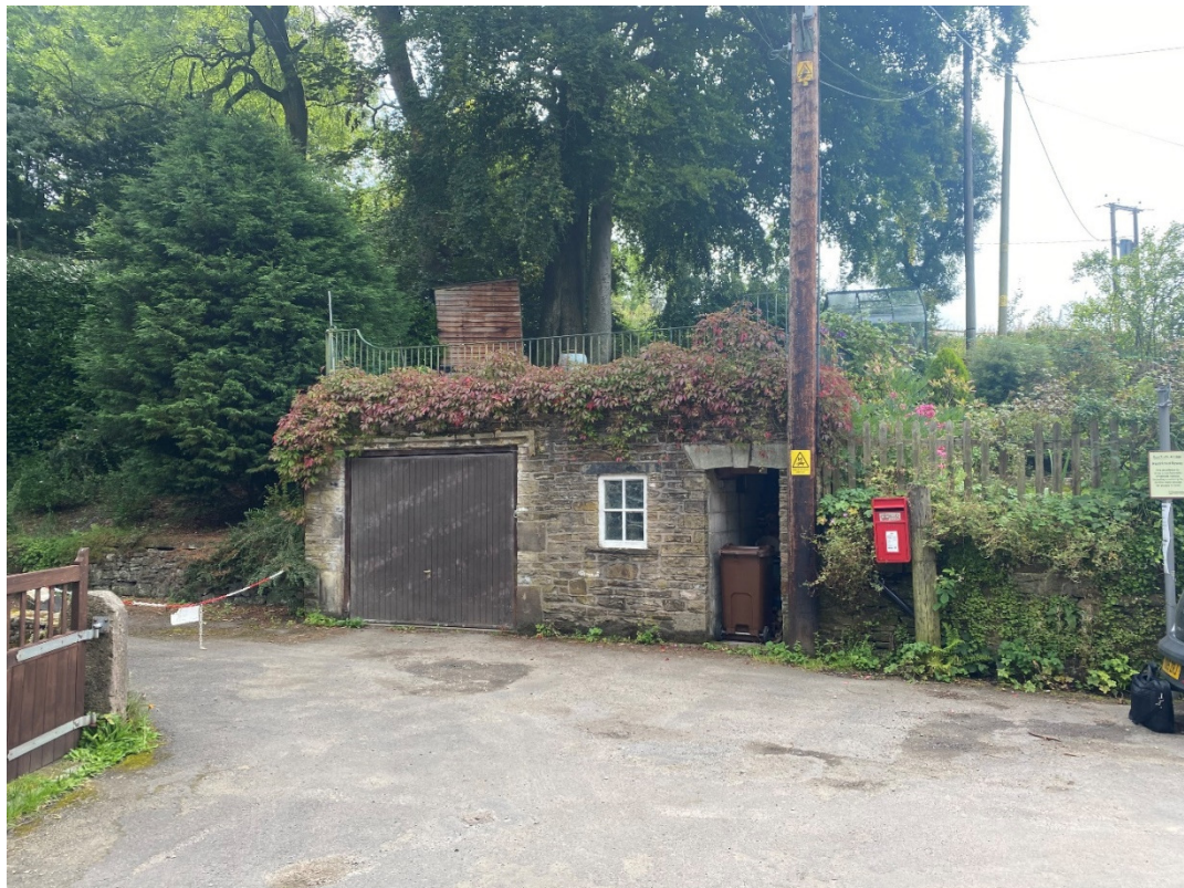
Detached Rivelin garage
