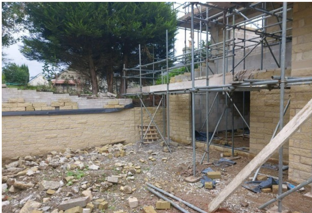
The approved construction is in progress
