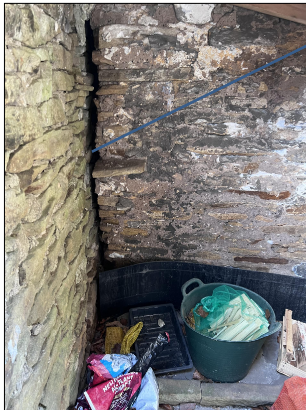
Figure 14: 'Shed 1' internal view showing internal wall joint with front boundary wall
