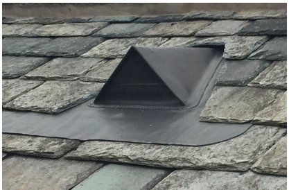
Example image of lead vent to pitched roof. N.B. Image not to scale.
