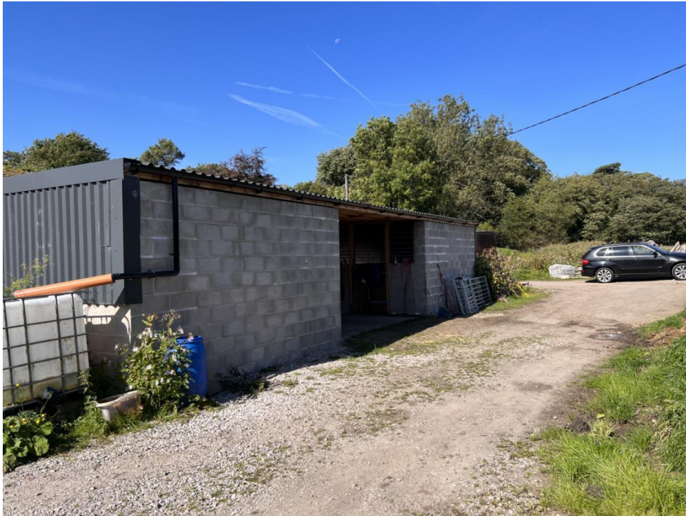
Figure 2: Northeast elevation of The Stable
