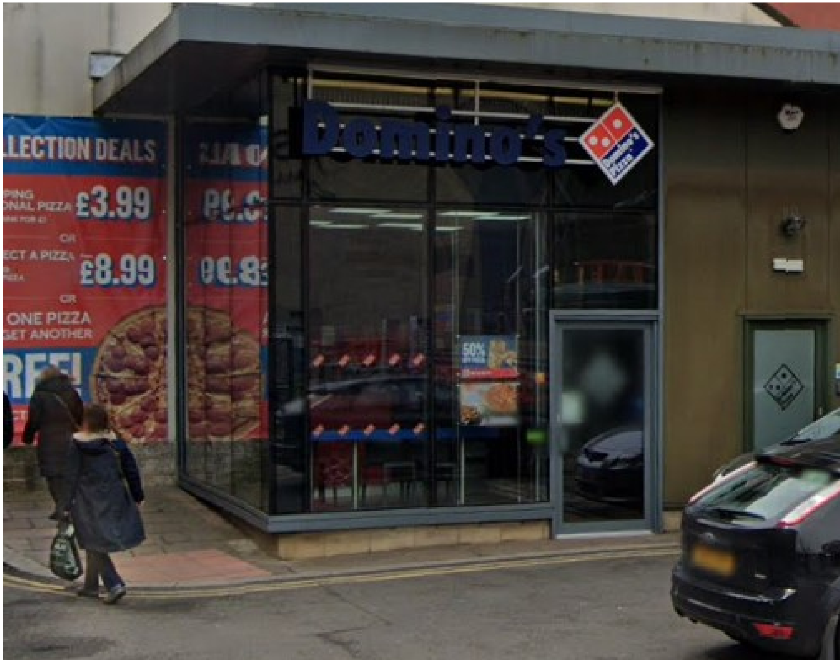
EXISTING REAR (EAST) PHOTO
