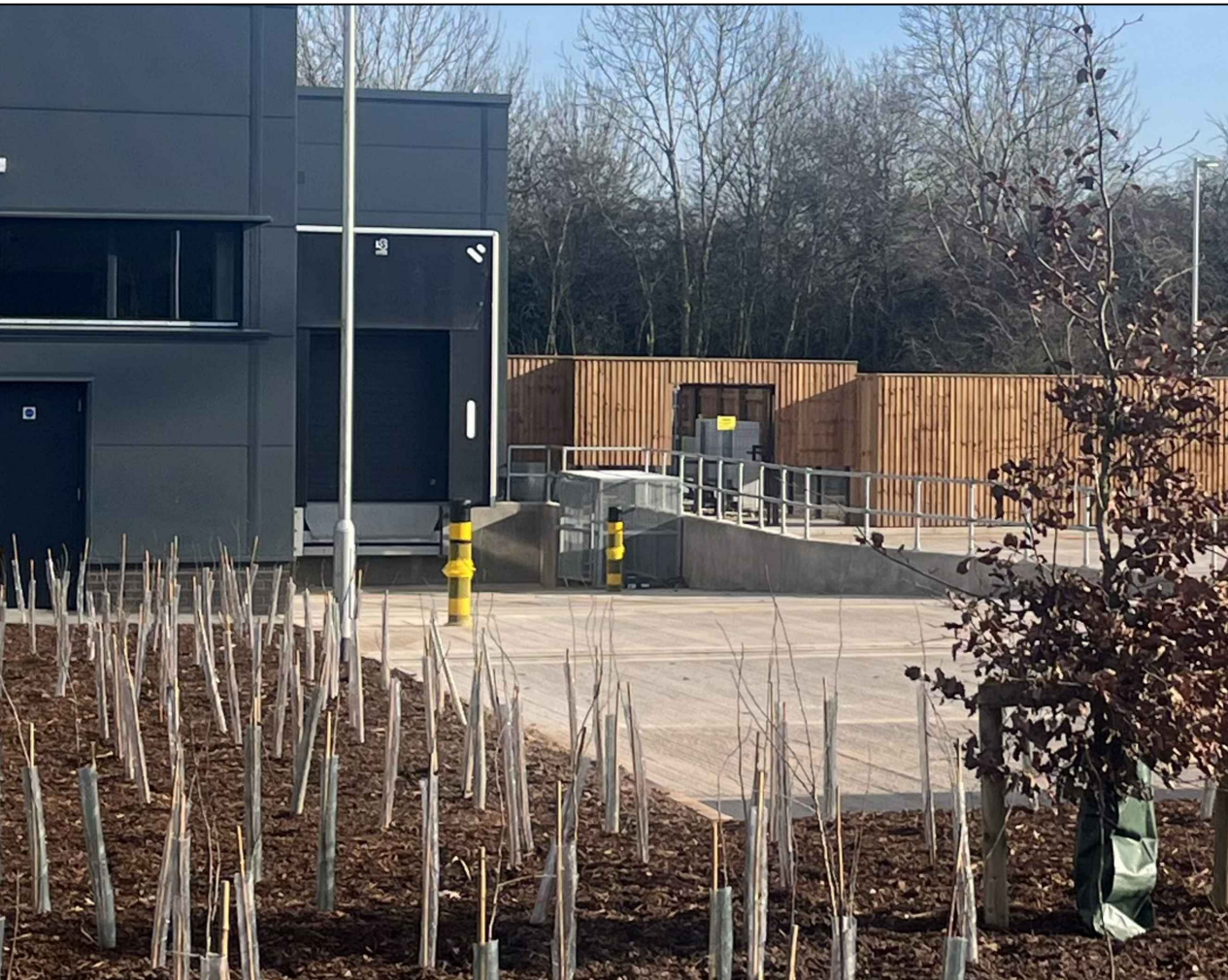
EXAMPLE: Delivery bay retaining wall at Aldi Battlefield
