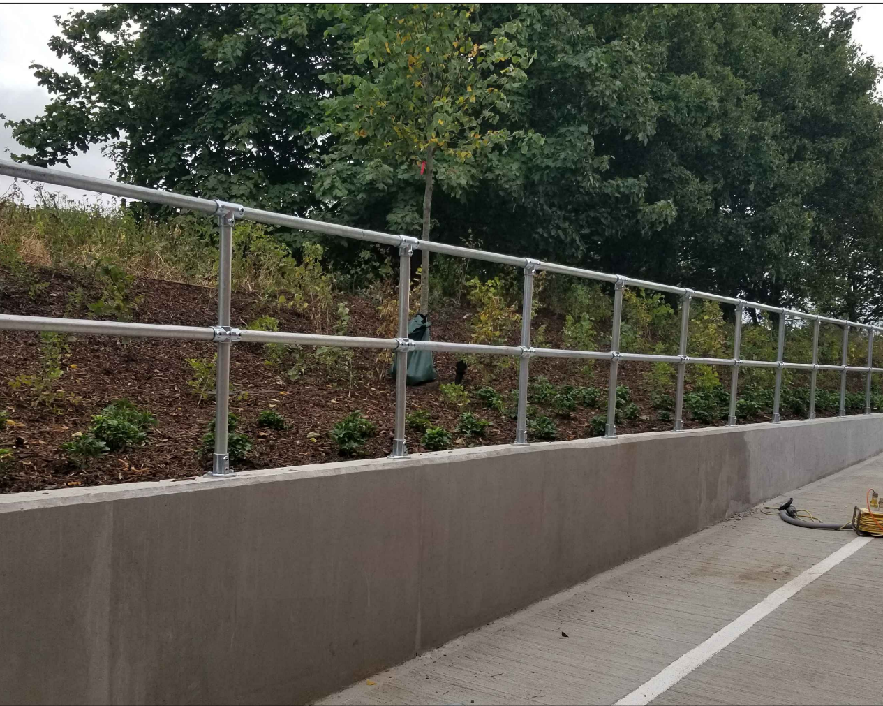
EXAMPLE: Delivery bay retaining wall at Aldi Tarleton
