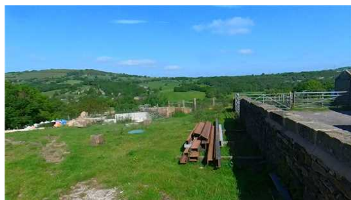
Existing UG LPG Tank
