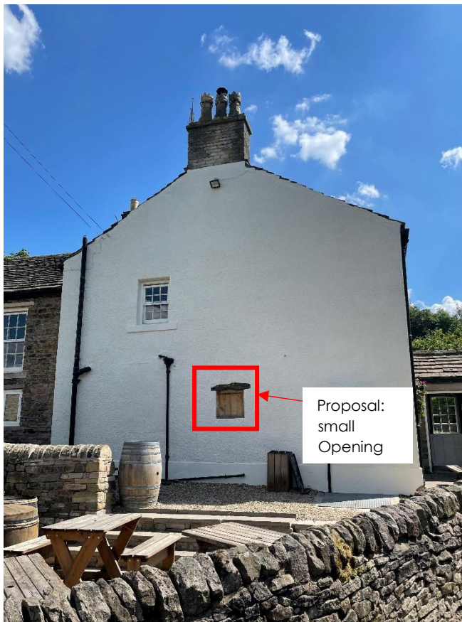
Figure 3: North Elevation showing extent of proposal – Insertion of 65cm (w) x 53cm (h) aperture within external rendered wall to form new opening. Located to the recess head level of the exposed infilled door (internally).
