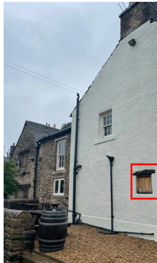
Figure 3: North Elevation showing extent of proposal – Insertion of 65cm (w) x 53cm (h) aperture within external rendered wall to form new opening. Located to the recess head level of the exposed infilled door (internally).
