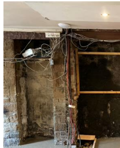
Figure 6: Existing opening uncovered during historic refurbishment of bar/servery. Existing doorway exposed when bar remodelling works were carried out some years prior.
