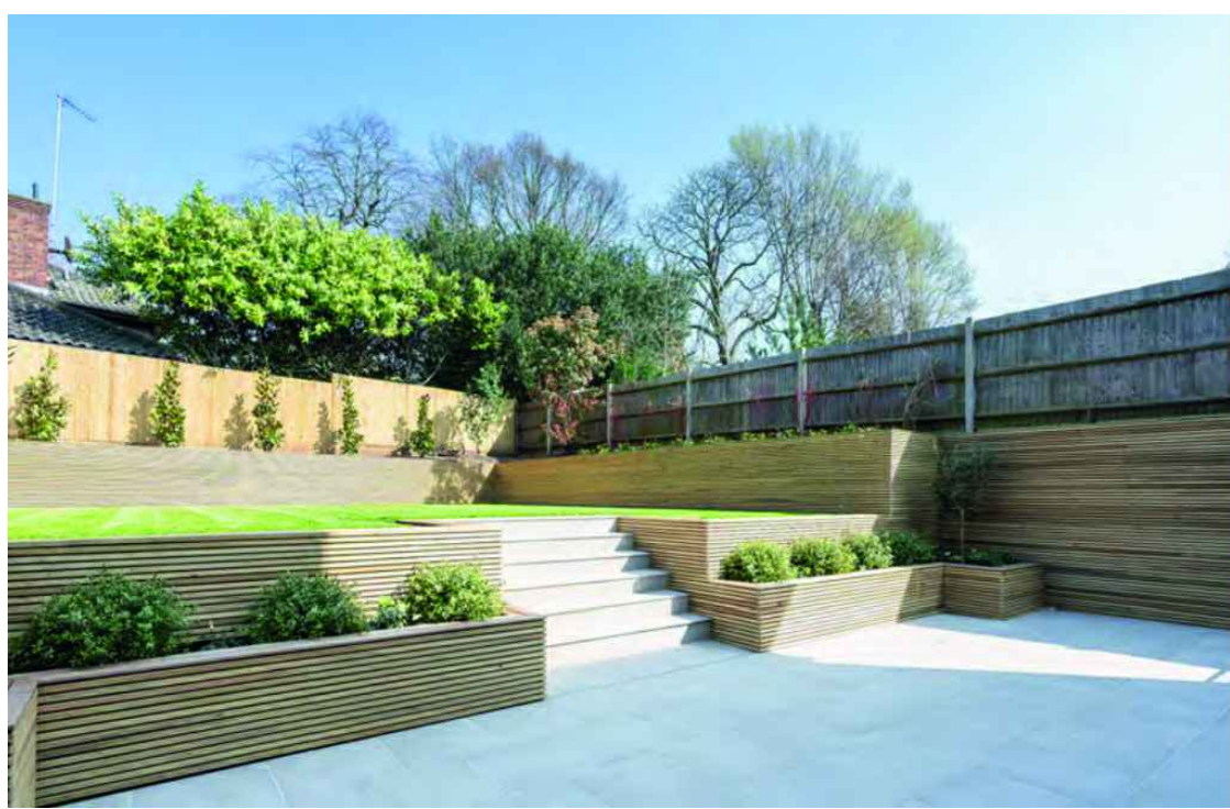
Cedar batten clad King Post retaining wall within rear gardens - Heights to be confirmed by the engineers.
