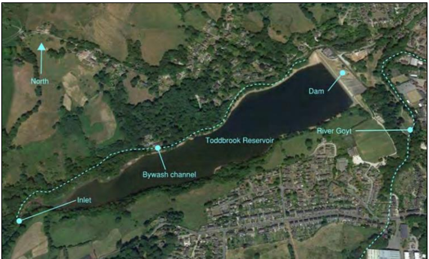
Toddbrook Reservoir – (fig. 01)
