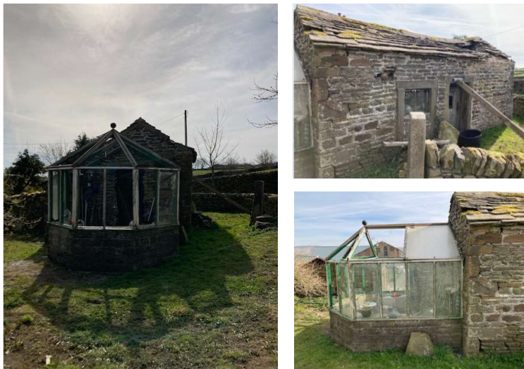
Left: Photographs of the stone outbuilding and attached conservatory/potting shed
