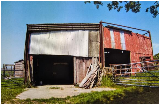
Figure 4: The original Agricultural Building on the footprint prior to deterioration.
