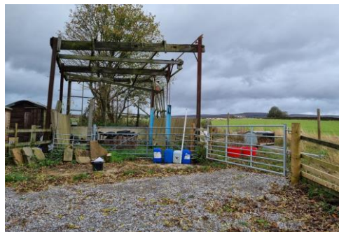
Figure 5: The remains of the Agricultural Building in November 2022.
