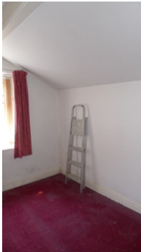
Sloping ceiling to bedroom window position with central exposed purlin.
