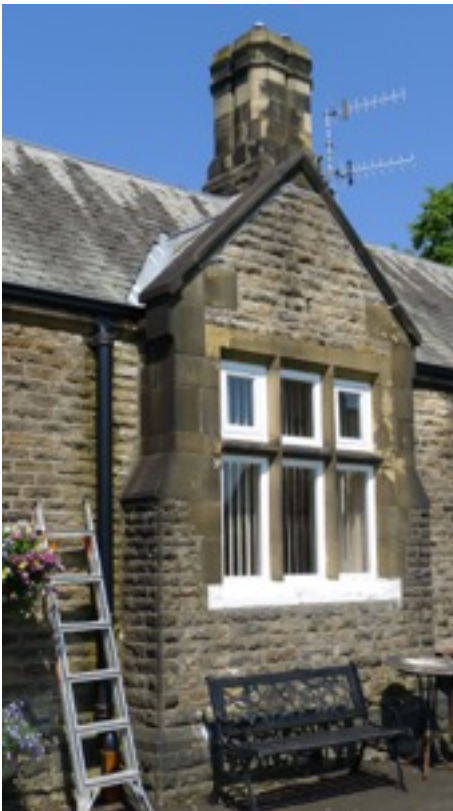
Gable bay window to the lounge in No.2
