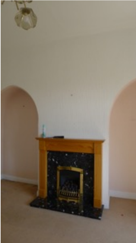
Arched niches either side of the chimney breast
