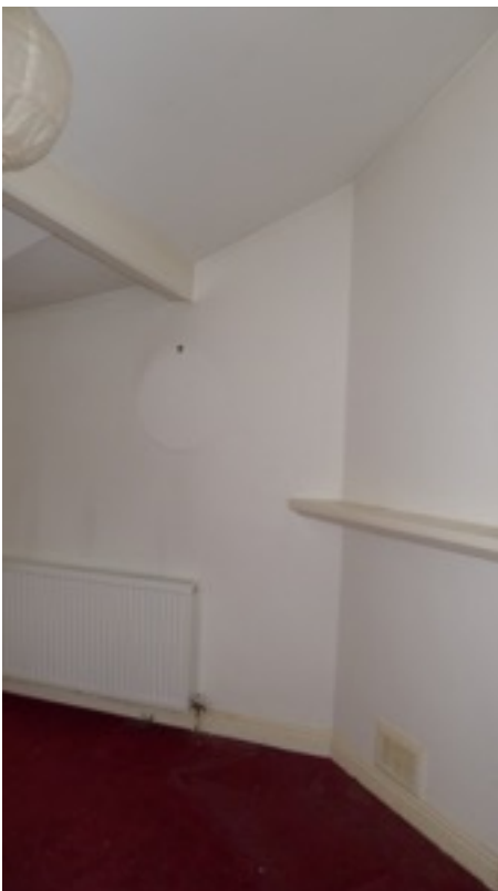
Sloping ceiling to former fireplace position.
