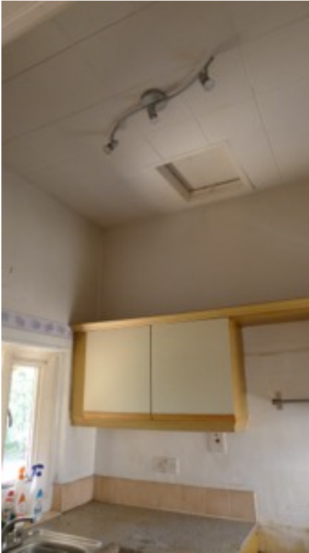
Polystyrene tiles to the ceiling and narrow loft hatch
