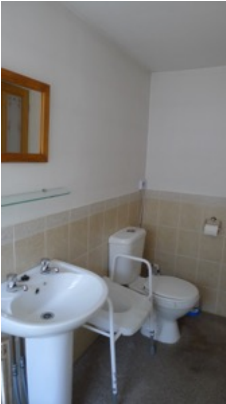
Existing sanitary ware, tiling and floor finishes to be upgraded.
