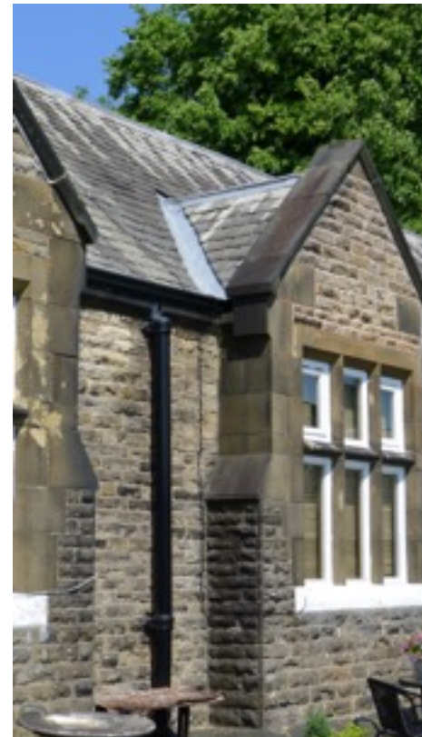
Gable bay window to the lounge in No.3
