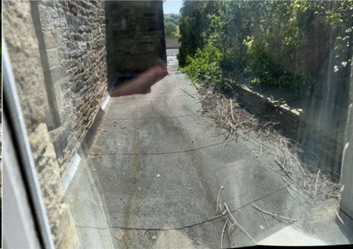
roof over kitchen, lantern to be inserted
