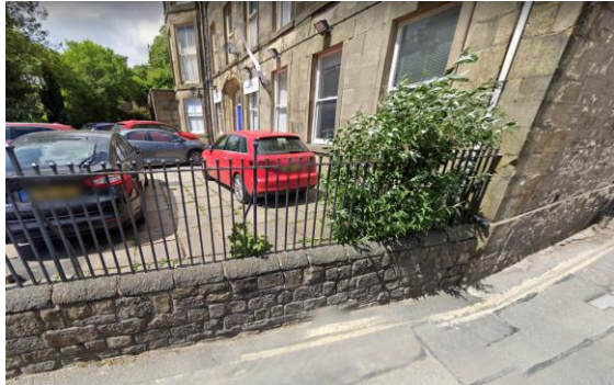
Existing railings adjacent to George Street
