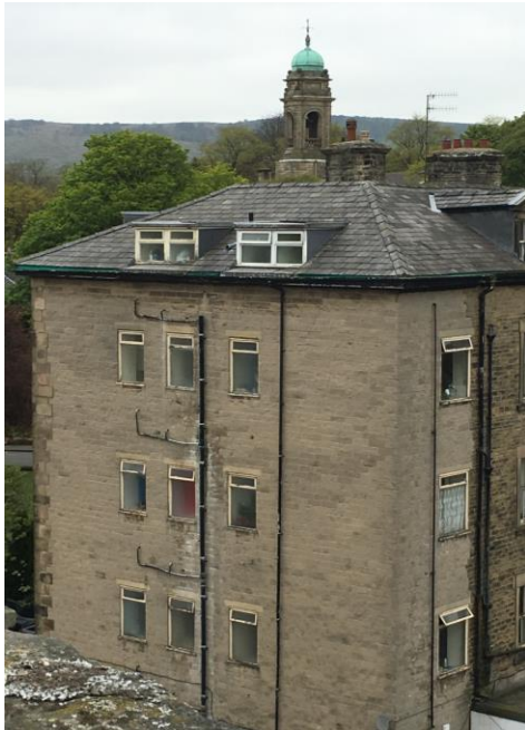
The existing facade is rather bland with large expanses of masonry
