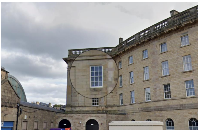
Mock window employed at The Crescent
