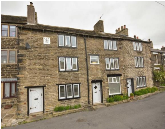
Fig.1 Photograph of front elevation
