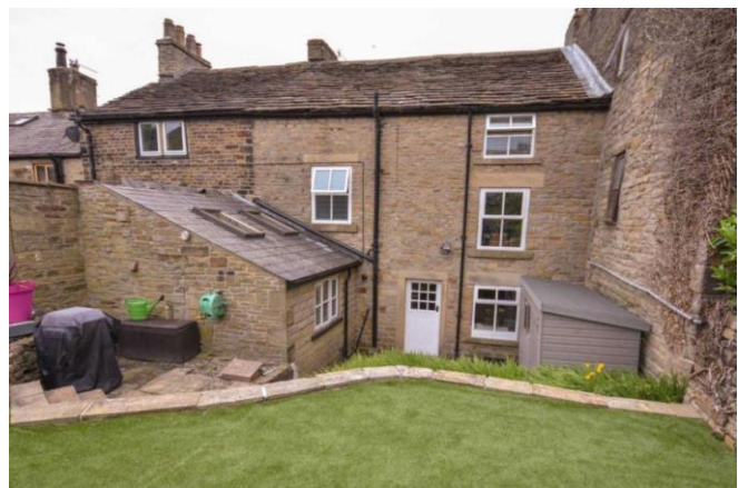
Fig.2 Photograph of rear elevation
