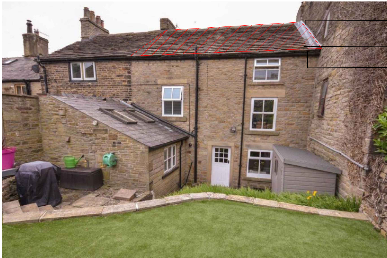
NORTH WEST ELEVATION - REAR PHOTO n.t.s
