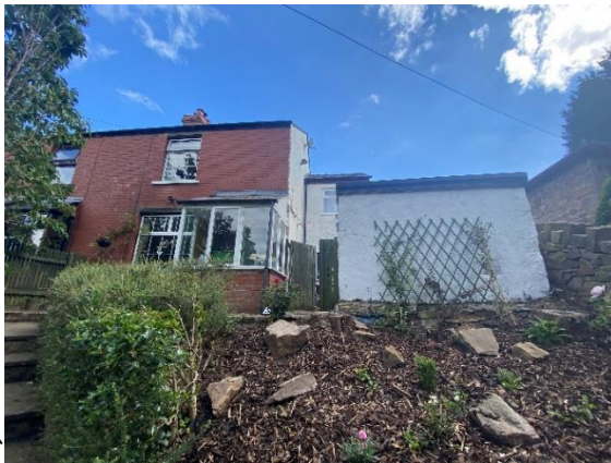
Fig.1 Front View of 150 Buxton Road
