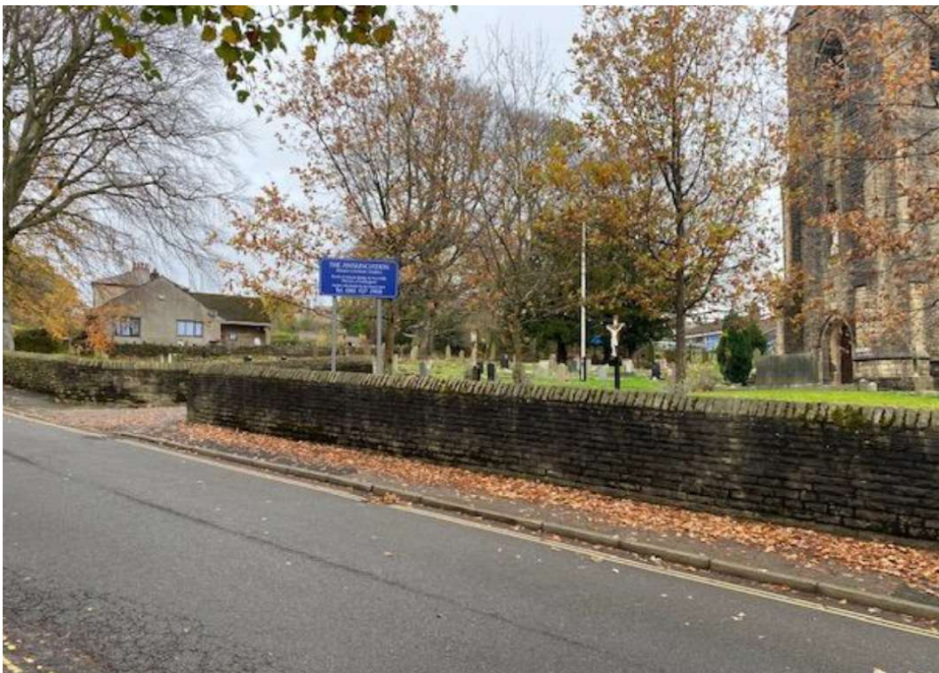
Figure 2: Gable end viewed from the south in the context of the church
