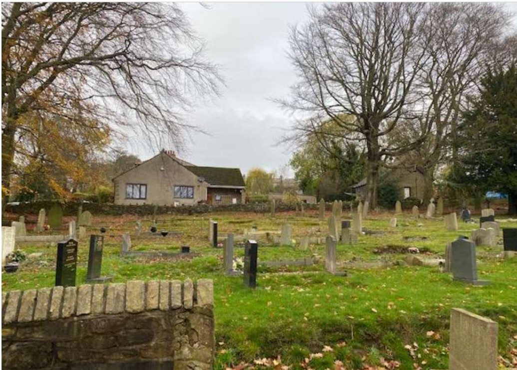
Figure 1: Gable end viewed from the churchyard
