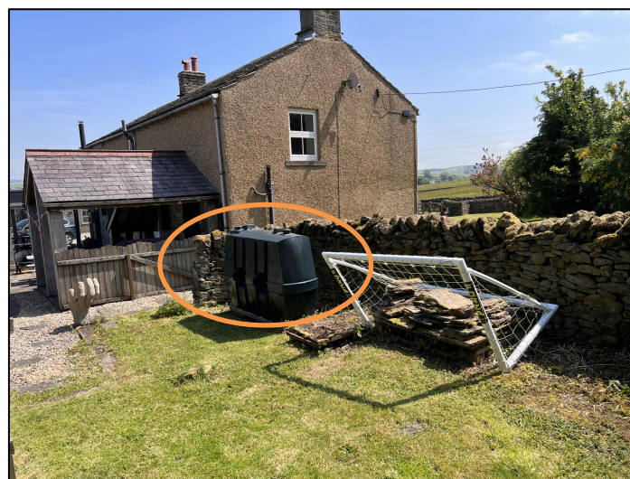
Figure 6: Oil Tank circled orange
