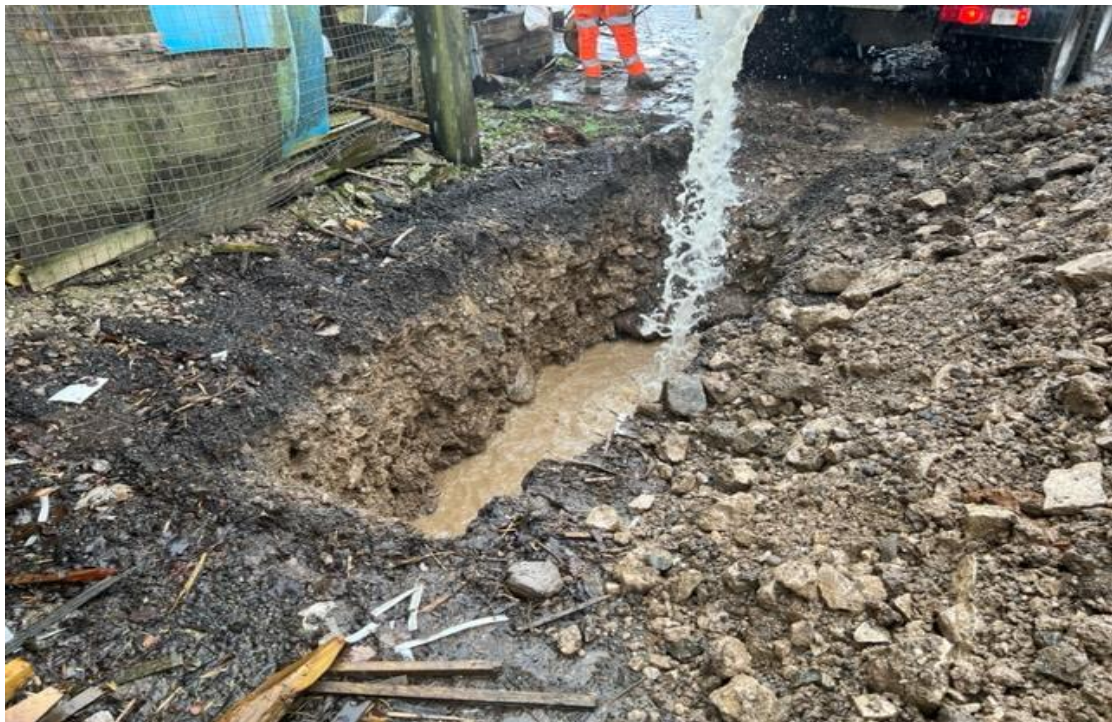
Excavation filled with water – water dropped immediately to the bottom of the gravel and cobble layer.
