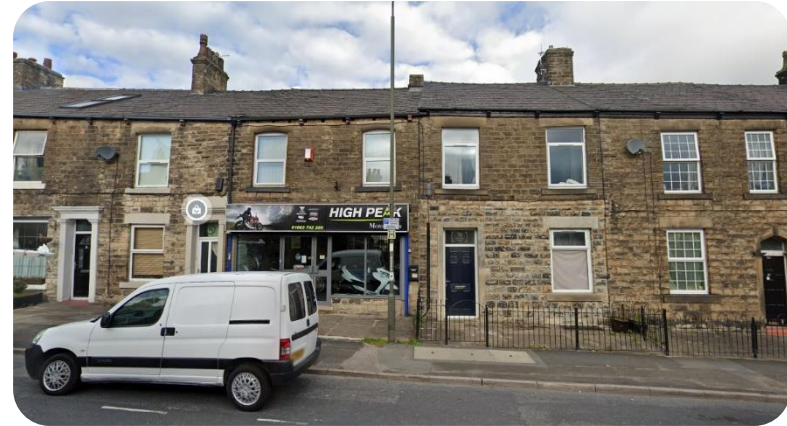
72 Albion Road New Mills
