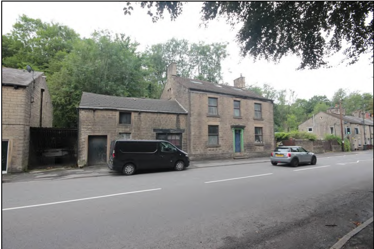
Photograph 8: View of the traditional buildings opposite Holy Trinity Church, on the southern side of Dinting Vale. Taken facing south-west
