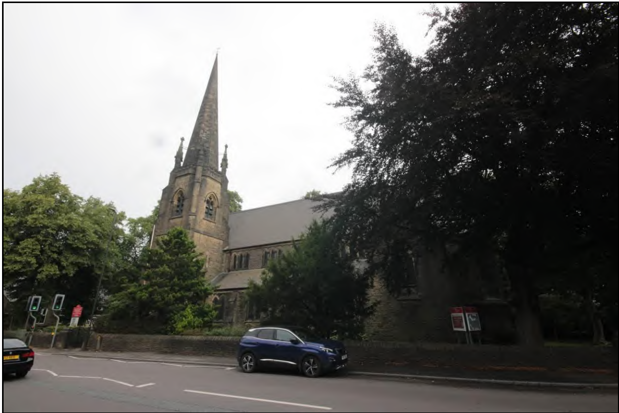
Photograph 1: View of the Grade II Listed Holy Trinity Church on Dinting Vale, taken facing north
