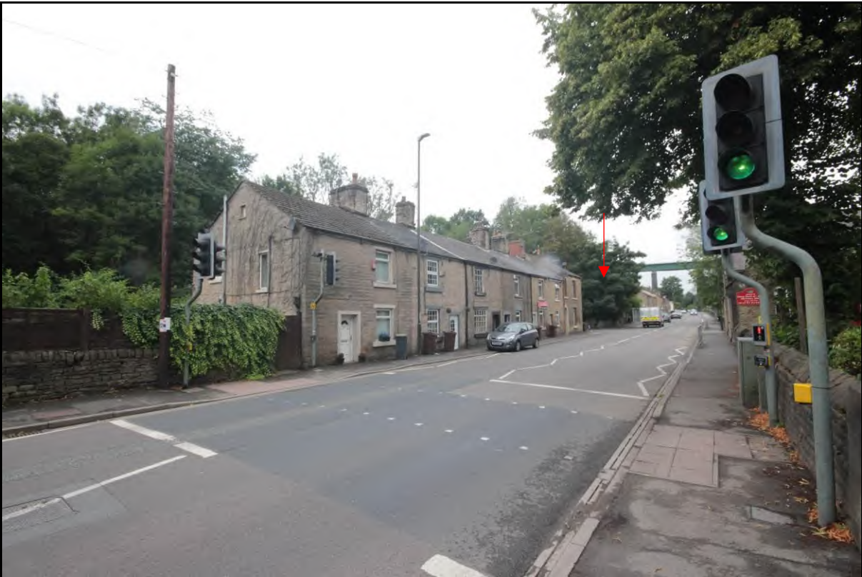
Photograph 19: View towards the proposed access point for the development on Dinting Vale (highlighted), taken facing south-west from Holy Trinity Church
