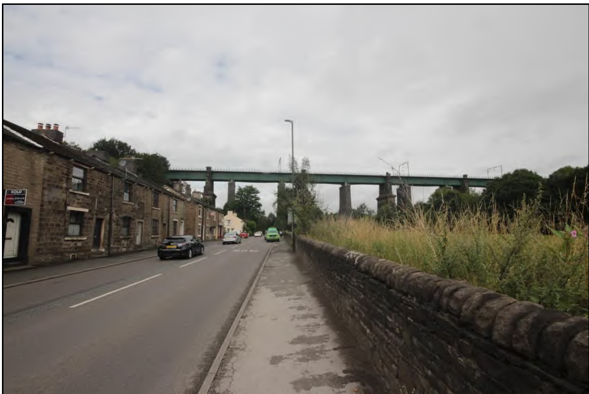
Photograph 3: View of the railway bridge to the north-west of Holy Trinity Church, taken facing north-west
