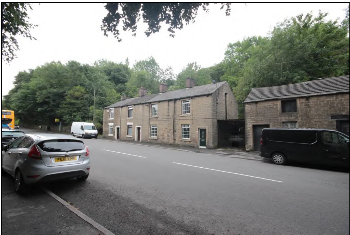
Photograph 7: View of the traditional terraces and cottages on the southern side of Dinting Vale, taken from the front of Holy Trinity Church facing south
