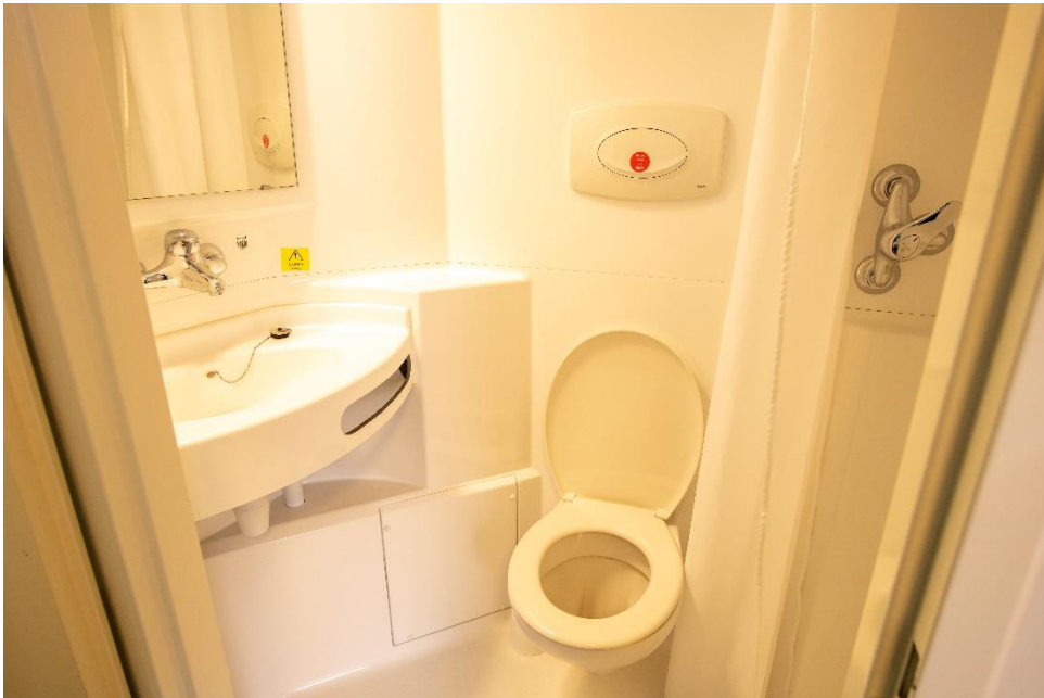
Ensuite shower room, within private bedsit room
