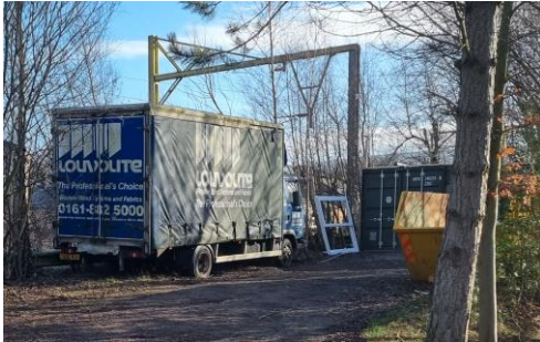
Figure 6: Area to receive the new unit viewed from the south west.
