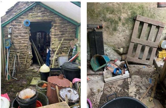
Left: Photographs of the interior of the stone outbuilding as set out under Appendix 6 of the Cover Letter
