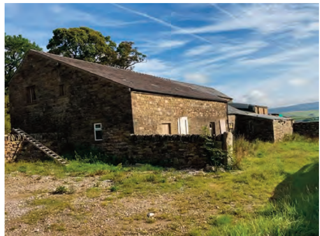
Highwood Farm Barn, South West Elevation.
