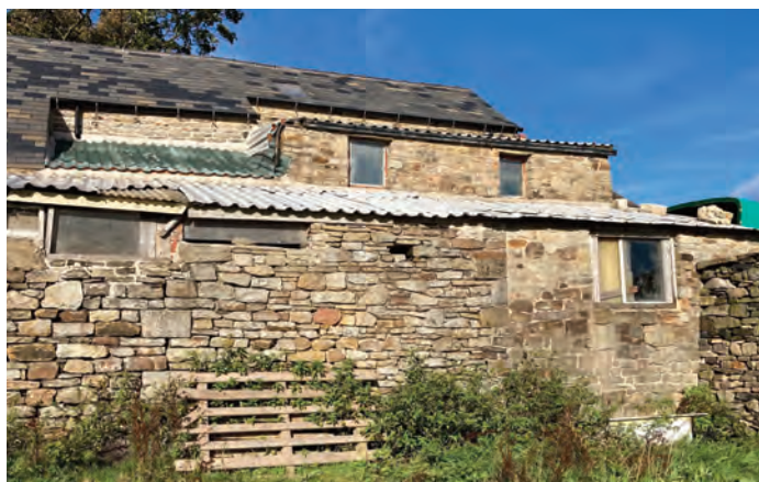
Highwood Farm Barn, Lean-to buildings South East Elevation.
