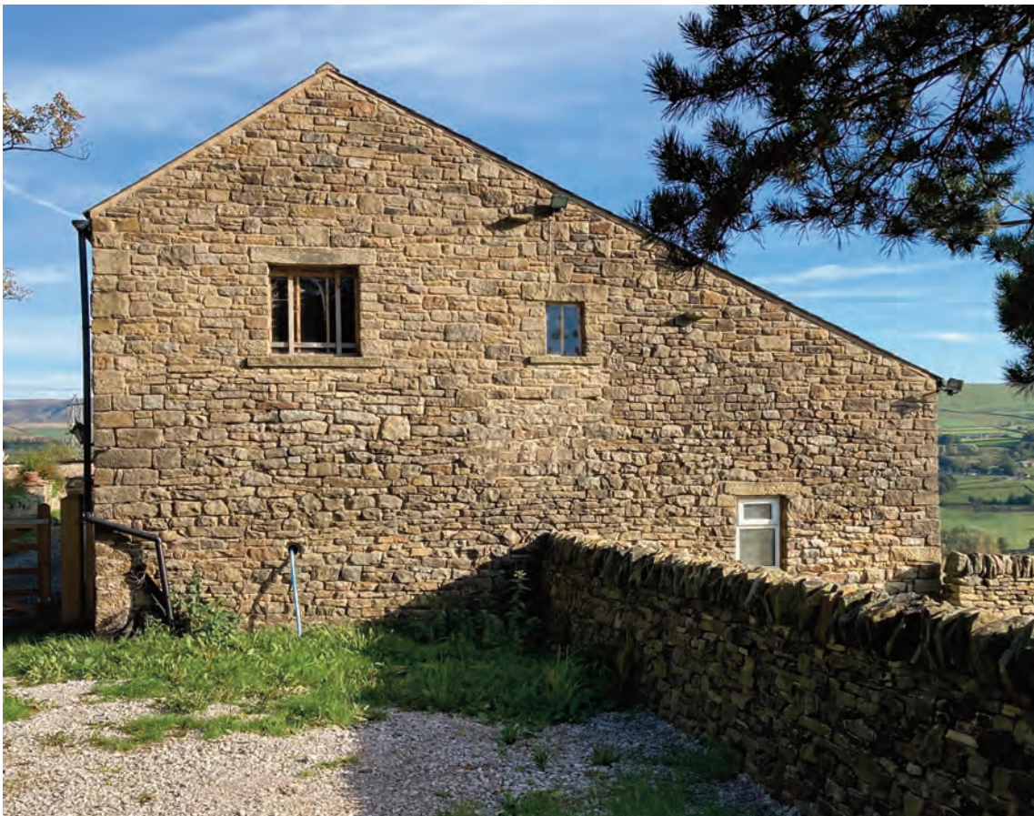
Highwood Farm Barn, West Elevation.
