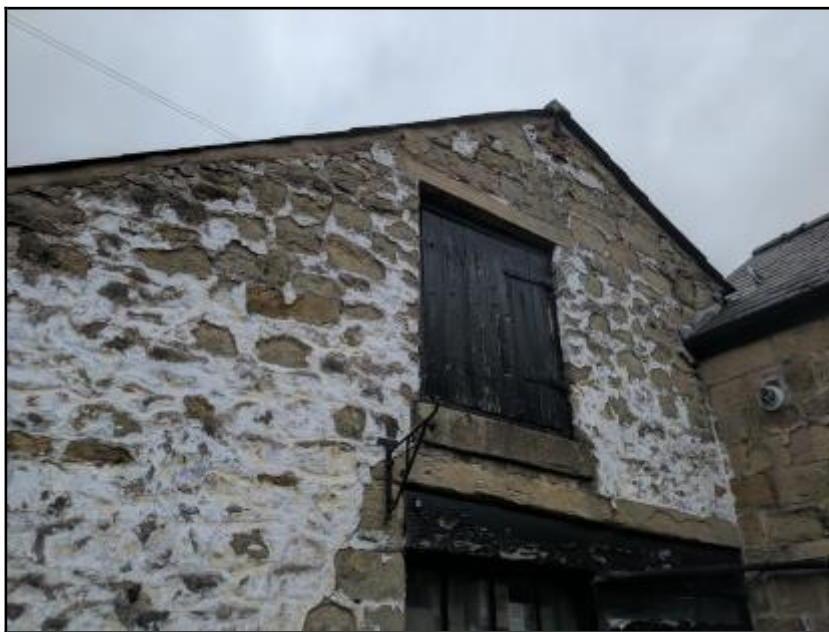
Photograph 9 showing the exterior of the shippon
