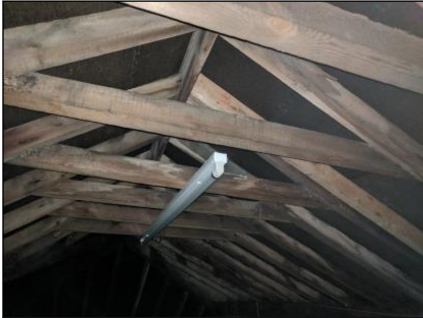
Photograph 12 showing the roof void of the shippon
