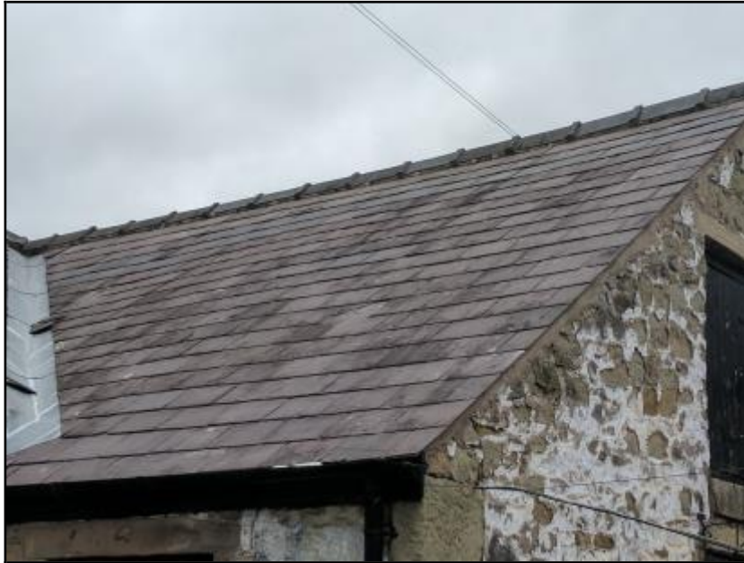
Photograph 10 showing the roof of the shippon
