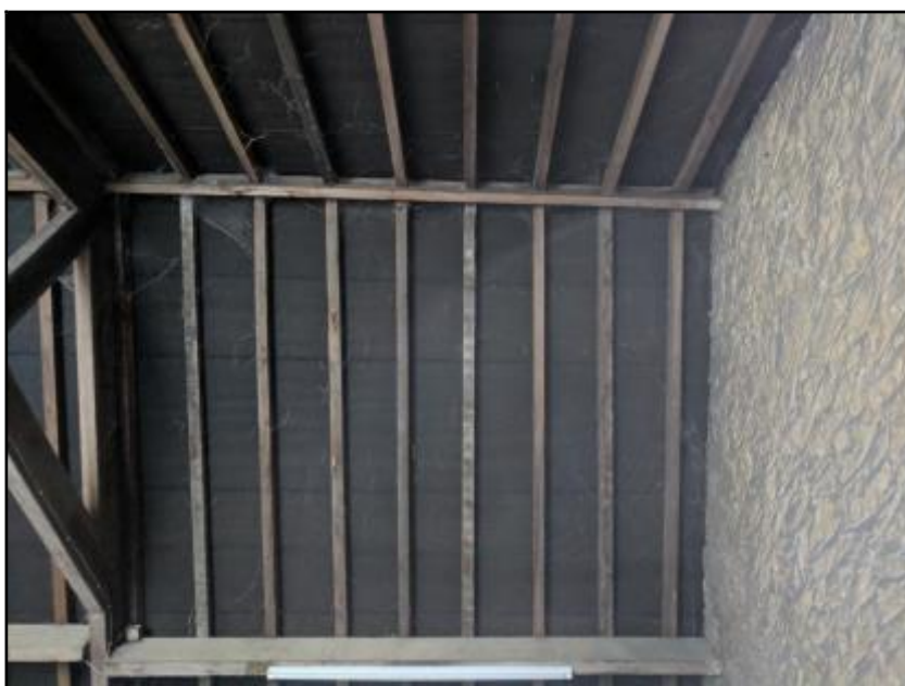
Photograph 13 showing the interior of the garages
