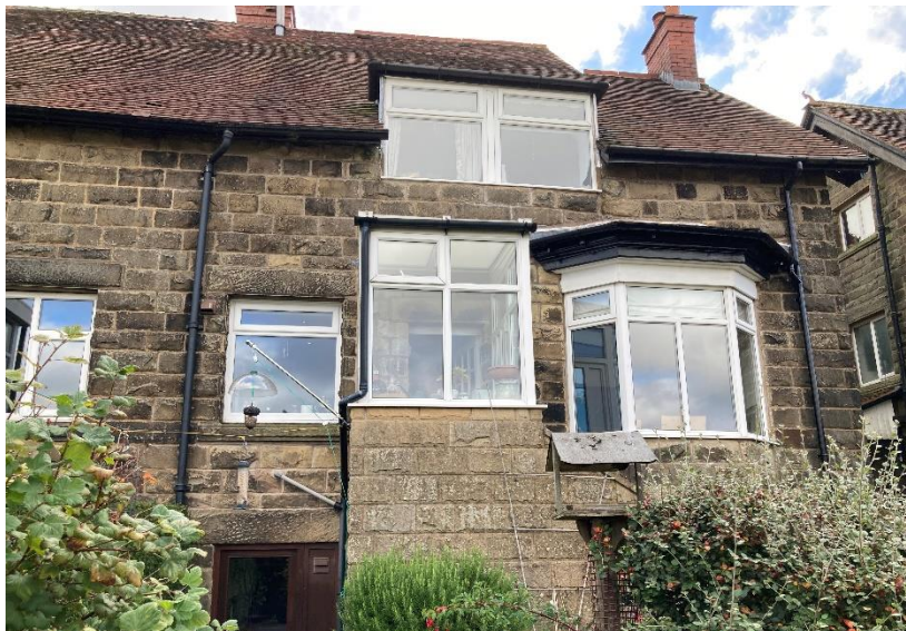
The current rear porch is not considered to be in keeping with the vernacular of the local conservation area
