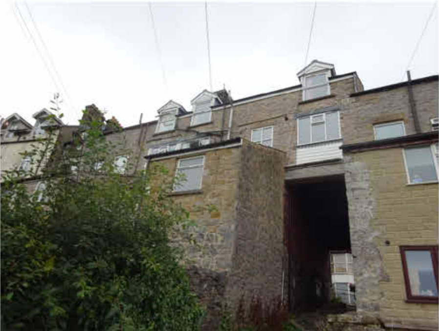
REAR ELEVATION PHOTOS
