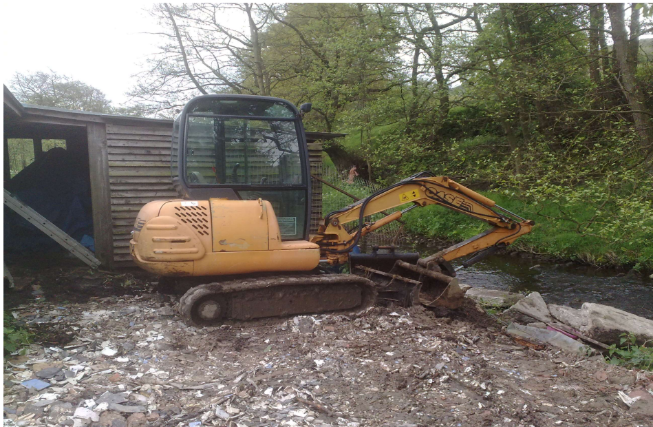
Excavator Parked Up 19 th May 2009
