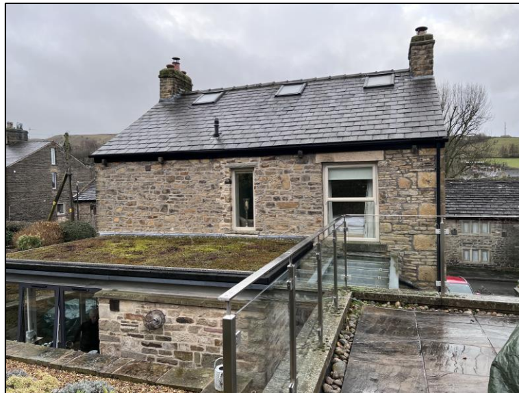
Figure 5: Northeast Elevation (rear).
