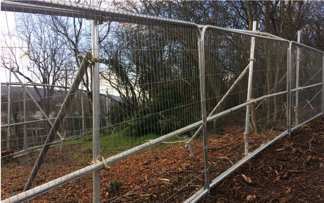
Above: Full specification barrier fencing.
