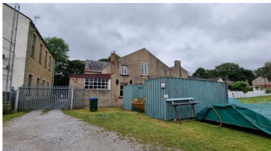
Figure 5: The rear of the site (eastern elevation) viewed from the cricket ground; the site boundary is on the line of the rear elevation with the shipping containers visible being the property of the cricket club.
