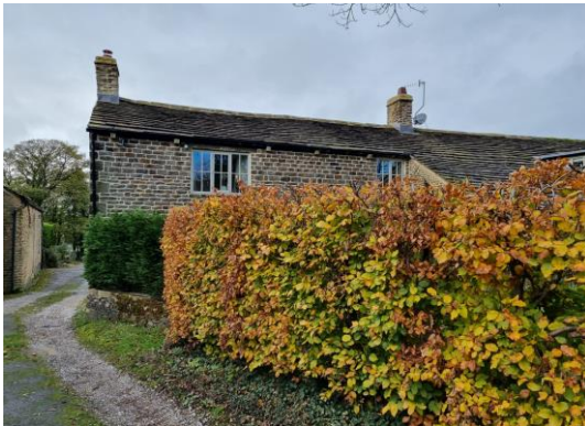
Figure 3: Rear elevation with Ground Floor obscured by hedgerow to south eastern boundary.
