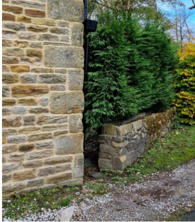
Figure 7: Existing boundary wall to the right of image and gable wall to the house to the left of the image.
