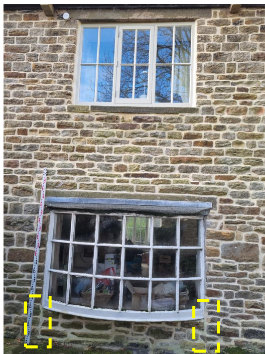
Figure 4: Rear elevation with bow window to Ground Floor and post-2018 window to First Floor
