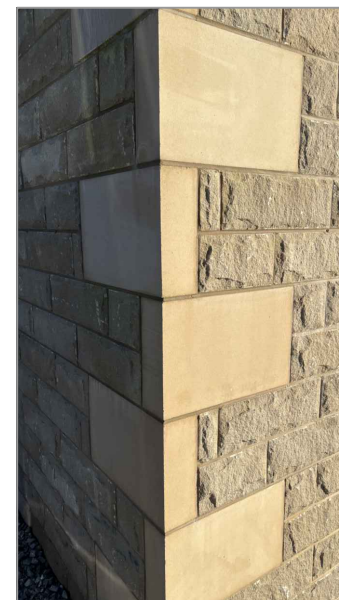
STONE DETAILING TO CORNERS AND CILLS ETC
