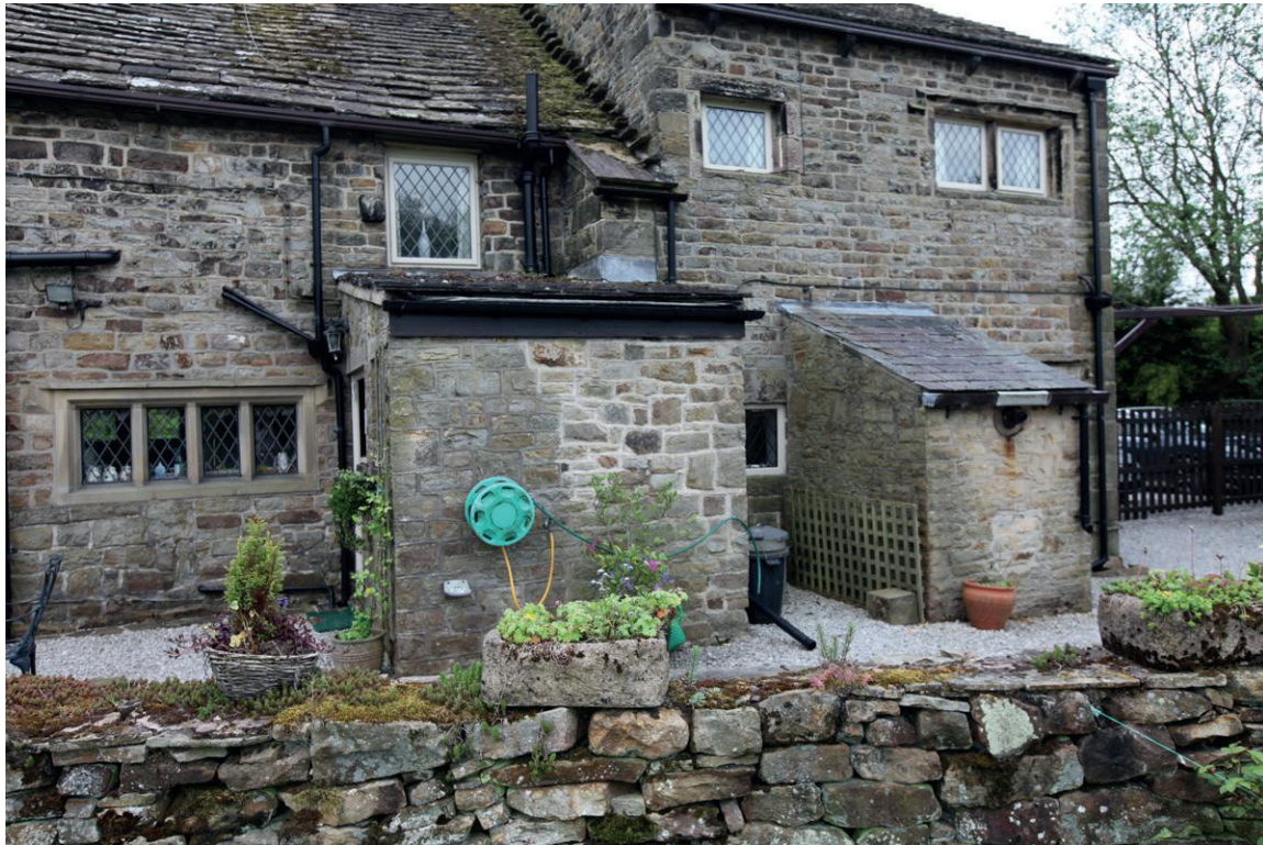
3. The north elevation with its small monopitched extensions and ad-hoc alterations
