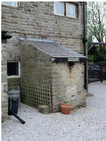
3. The north elevation with its small monopitched extensions and ad-hoc alterations
