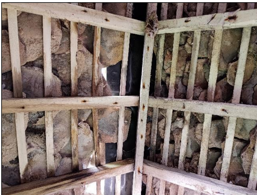
Photograph 6 showing the roof structure of the upper floor
