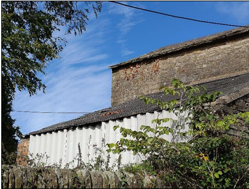
Photograph 4 showing the lean-to
