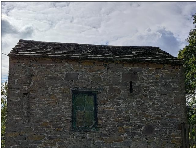
Photograph 3 showing the roof of the property
