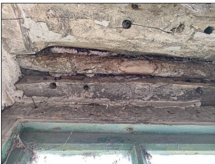
Photograph 7 showing the window lintel
