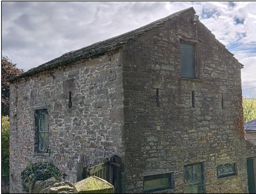
Photograph 2 showing the exterior of the building from the rear
