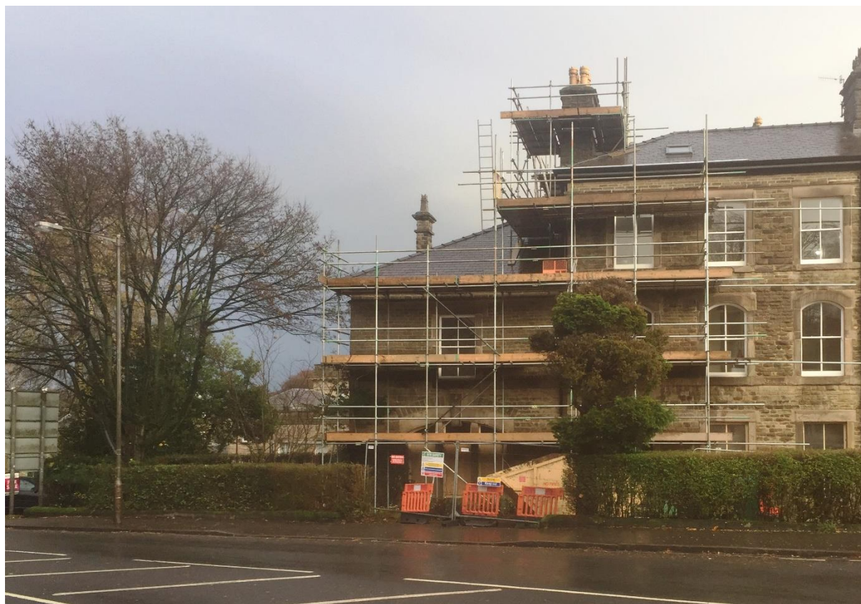
Area of land for bin store (photos with and without annotation)
